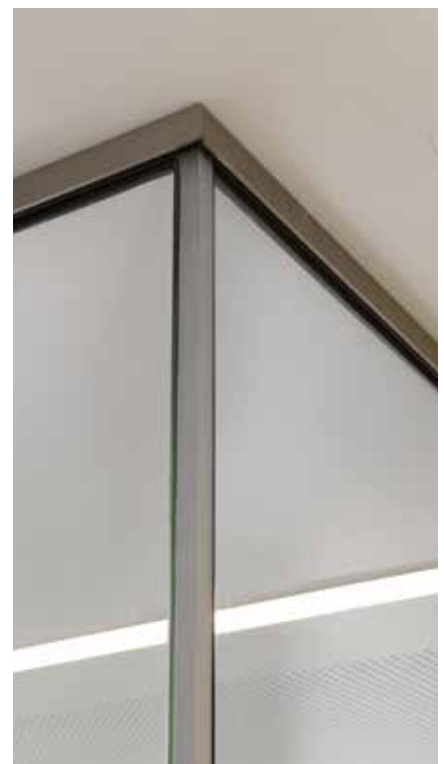
DETAIL E CLIP-IN H-profiel™
